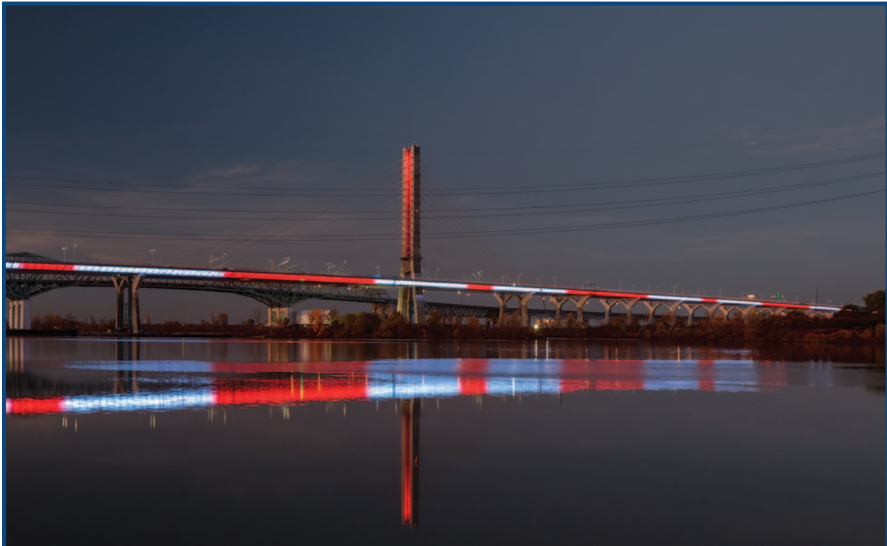
The system covers four miles, two miles per side, with 7,606 fixtures and 22,818 control parameters, or 45 universes of control parameters across 189 different universes. The project consumes 380,000W.
